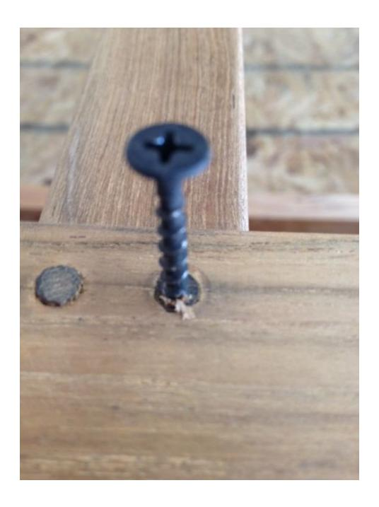
Then, using a claw hammer, or pliers (hammer is easier), grab a hold of the screw head and, while resting the hammer head against something to prevent damaging the wood, pry the dowel from the dowel hole.
